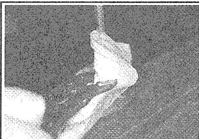
Fig. 19 This locknut was removable using a locking pliers and a shop cloth (to protect the chrome nut). Unscrew the locknut to remove it
